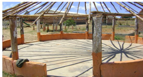
Insaka repairing in progress
