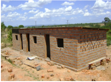
Chicken run underway
